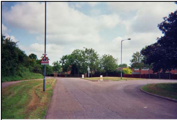
Typical view – main road
